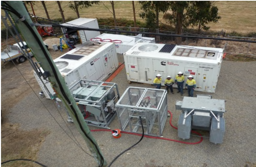
CTX Unit – Caged transformer, NULEC recloser and generator
