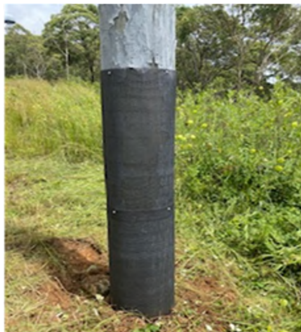
Figure 8 - Install Pole Wrap
