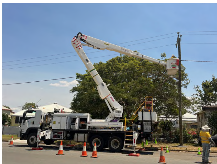
Figure 1: Example EWP in operation
