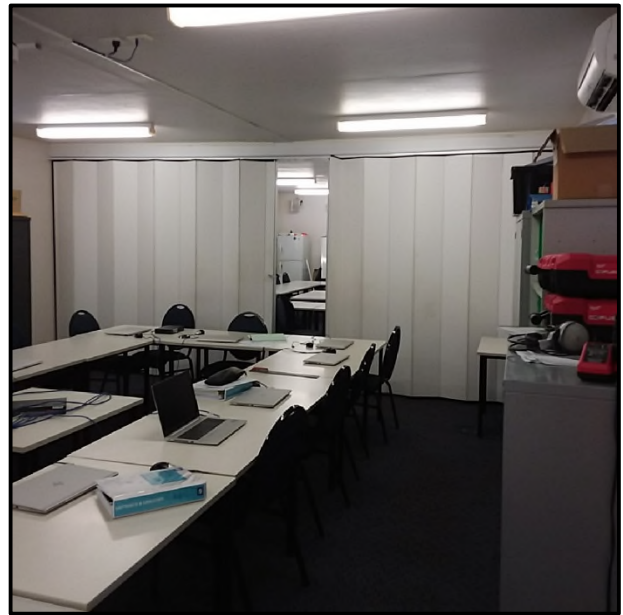
Block 8 – Internals (note: constrained space, old curtain wall, inefficient lighting & A/C)
