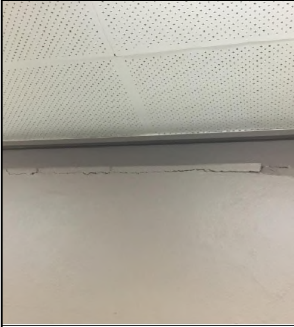
Building A – Movement & cracking to rendered capping
