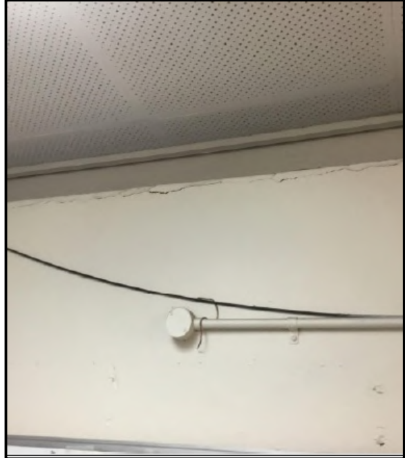
Building A – Continued movement & cracking to wall
