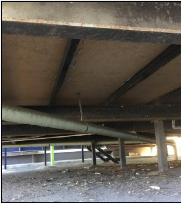
Training Demountable – Underfloor, plywood on steel frame
