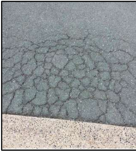
Yard Surface – Bitumen crocodile cracking
