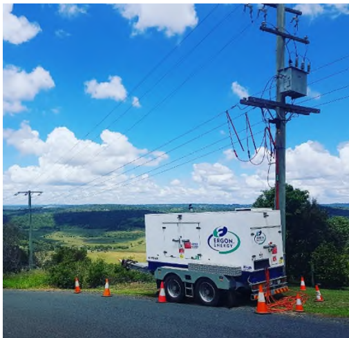
CTX Unit – Caged transformer, NULEC recloser and generator
