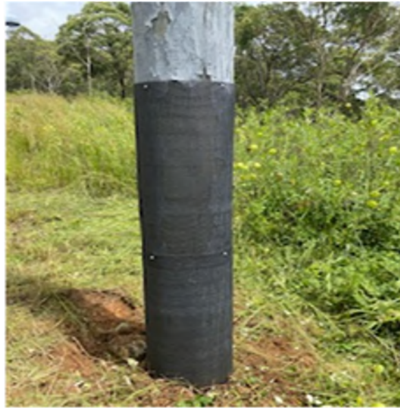
Figure 8 Install Pole Wrap
