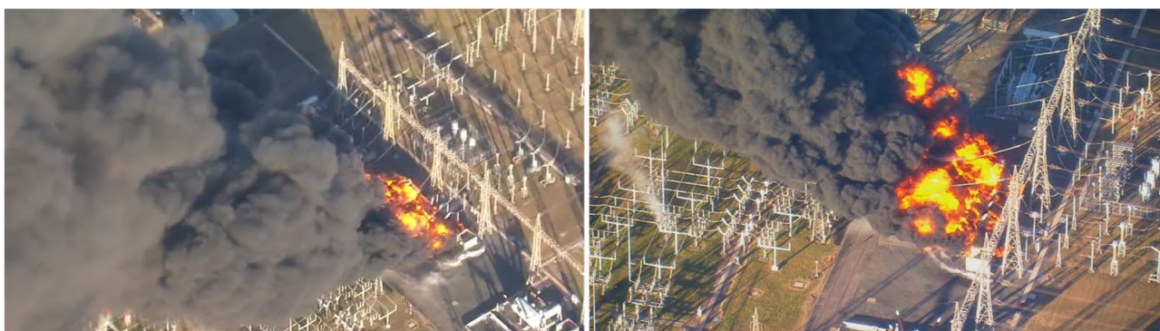
Figure 5-2 Photos of Dapto Substation fire 8
