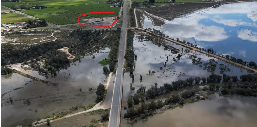
Figure 10 - Renmark zone substation and flooding adjacent.
