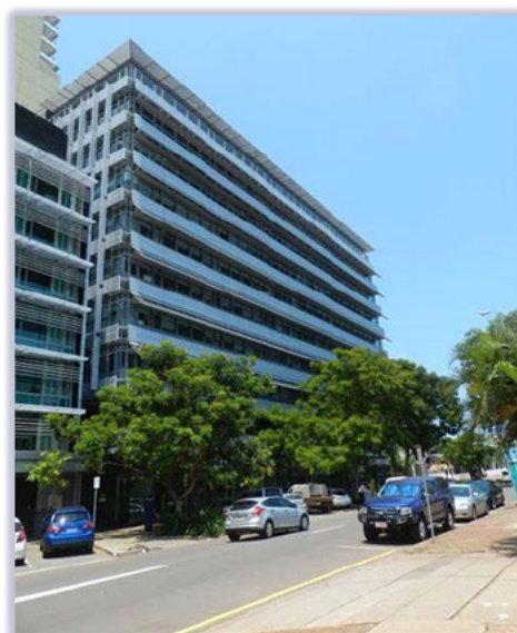
Figure 2 – Jacana House (Tower)
