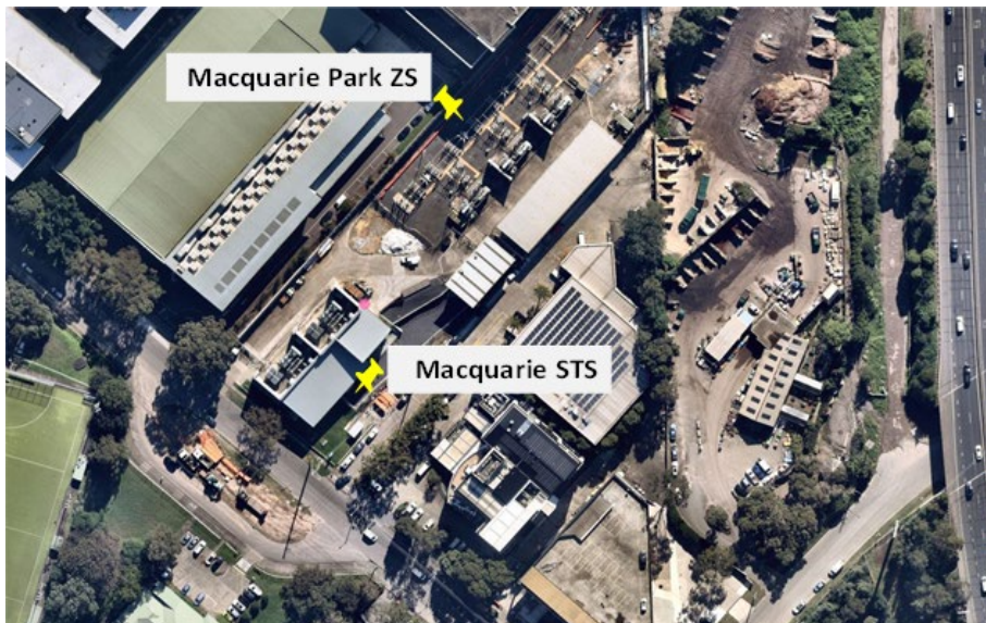
Figure 5. Overview of Macquarie STS and Macquarie Park ZS site
