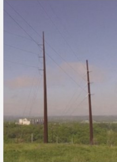
NEW MONOPOLE STRUCTURE
