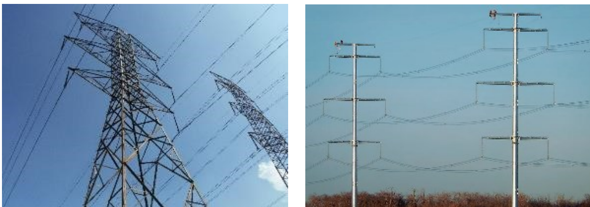
FIGURE 1: TRANSMISSION INFRASTRUCTURE, LATTICE VS MONOPOLES
