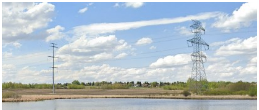
FIGURE 2: MONOPOLES USED IN 10KM OF TRANSMISSION LINE TO GAIN COMMUNITY SUPPORT
