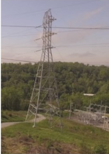
EXISTING LATTICE TOWER STRUCTURE
