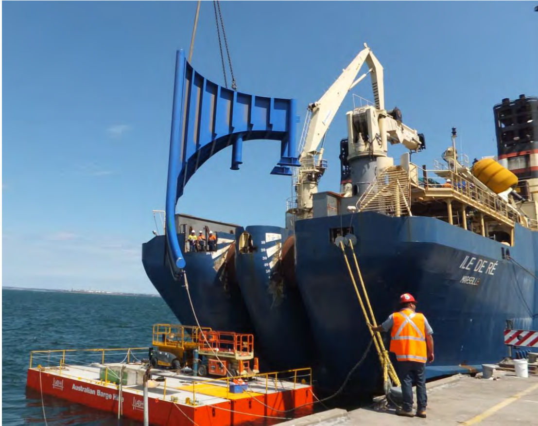
Figure 7.5 - A cable chute being fitted to the Ill De Rae
