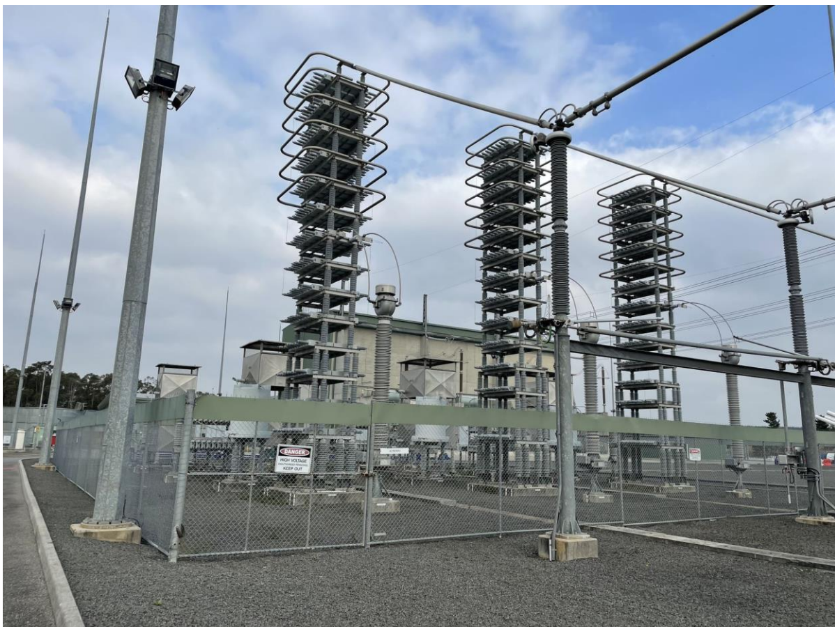
Figure 2.3 Basslink's AC filters
