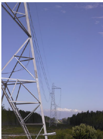
Figure 20. Overhead line Overview
